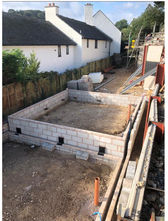
The first foundations
