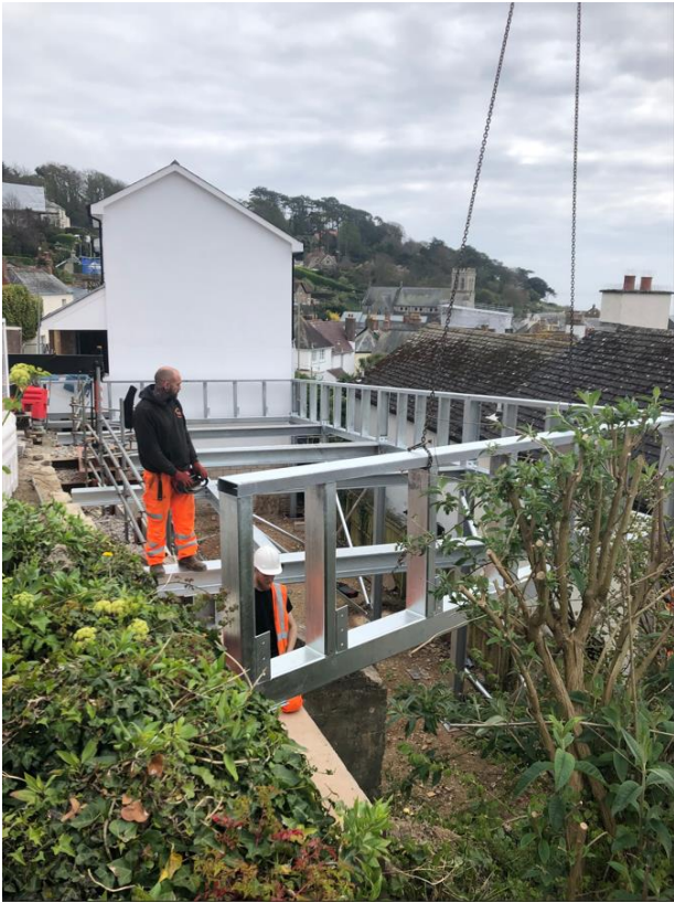
Car park decking and house No 1
