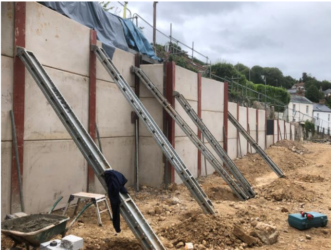
The new retaining wall
