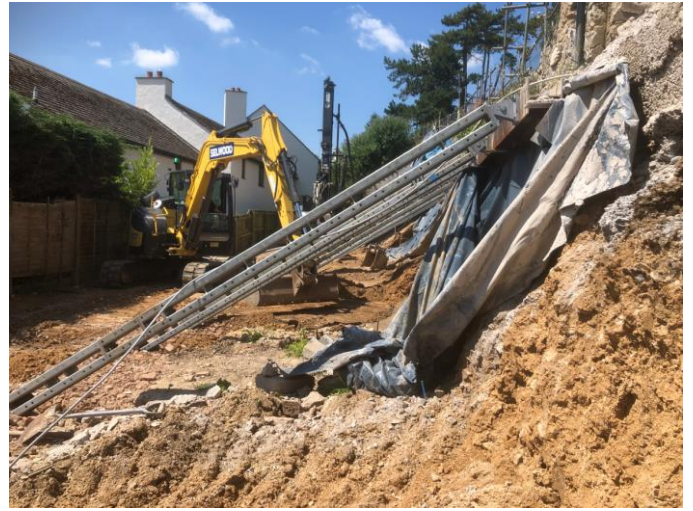
Constrained site work
