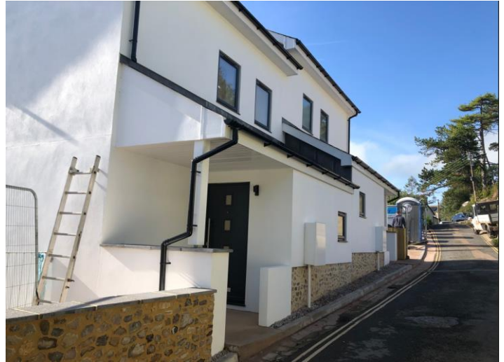
View up Berry Hill before completion showing flint walling
